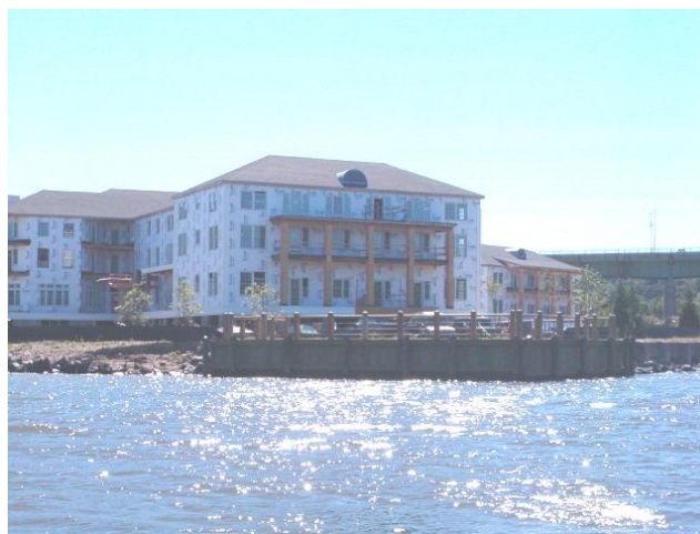
Work at Sterling Glen in Roslyn, October 2006 (photo by Carol DiPaolo)
